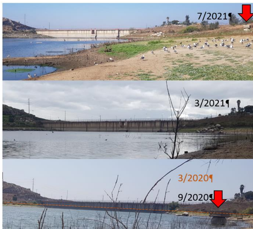
Figure 7. Pictures of the southern wall of the Ensenada Reservoir ("Presa Emilio López Zamora"), that documented the water level variation. The orange line indicated the water level observed in March 2020 and marked in the wall. The red arrow indicated a cement permanent structure, as a reference of the water level.
